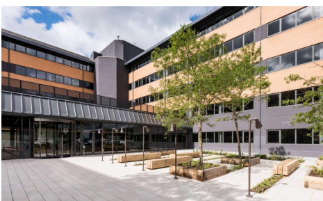
Reception Entrance (Ground Floor)
